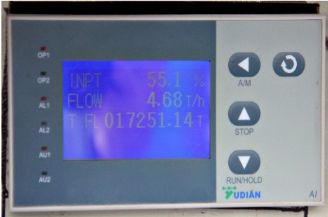
Steam Flow Meter Installed
